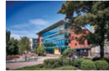
Ambika Paul Building
